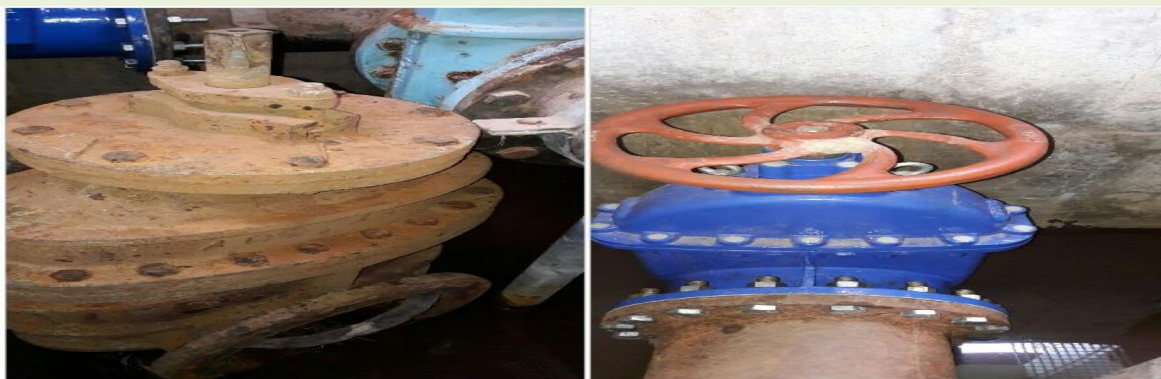
Replacement of old Valves at 7ML Reservoir
